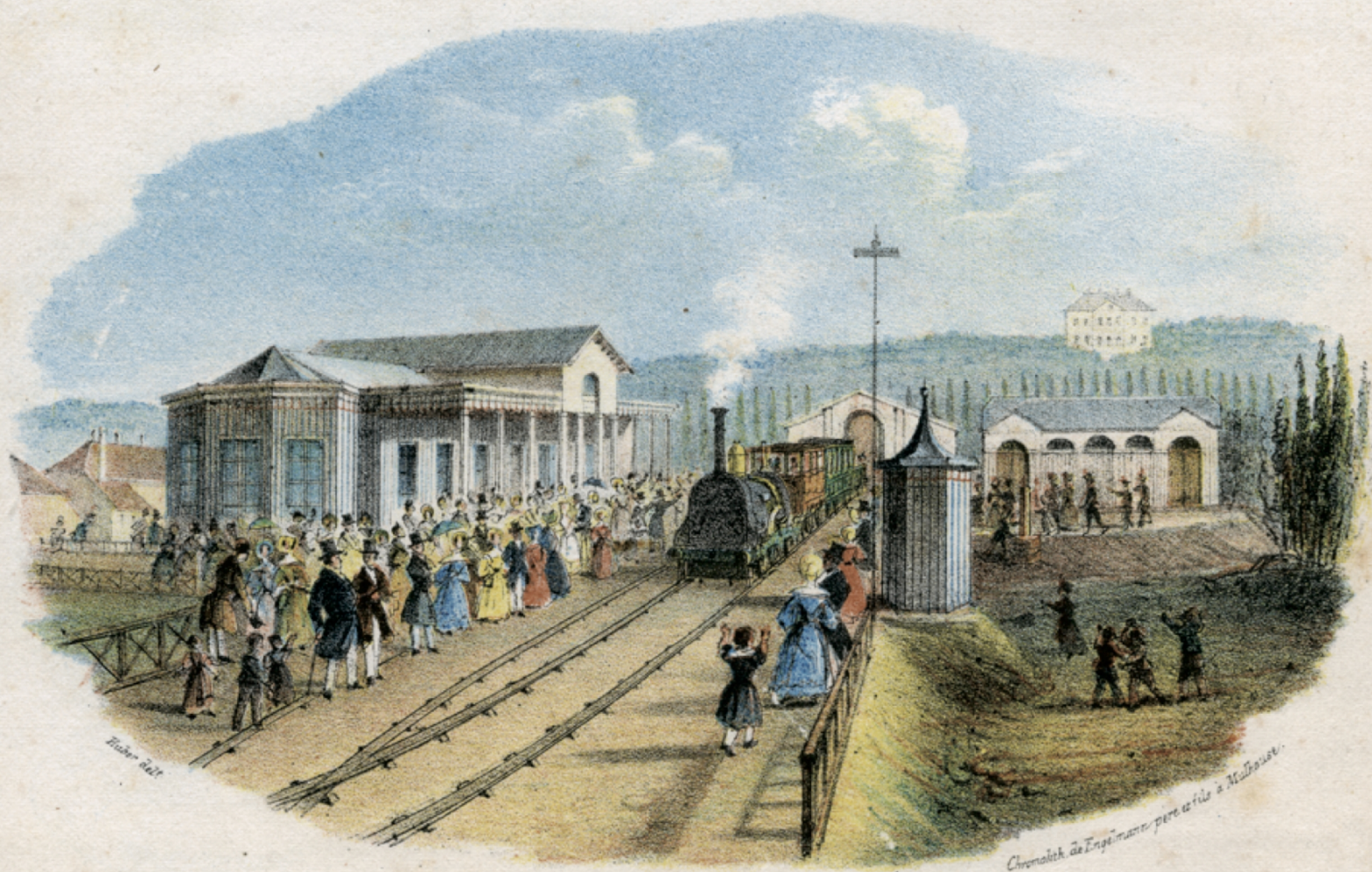
Station provisoire de Mulhouse.
