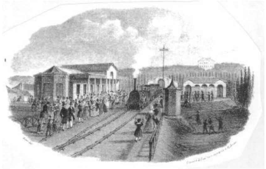
Station provisoire de Mulhouse
